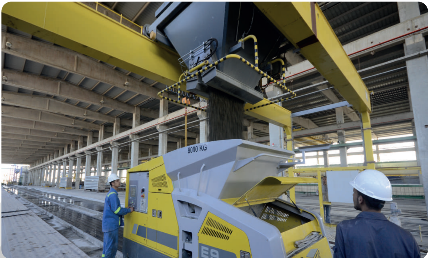
Automatic concrete feeding by flying bucket & hooper
