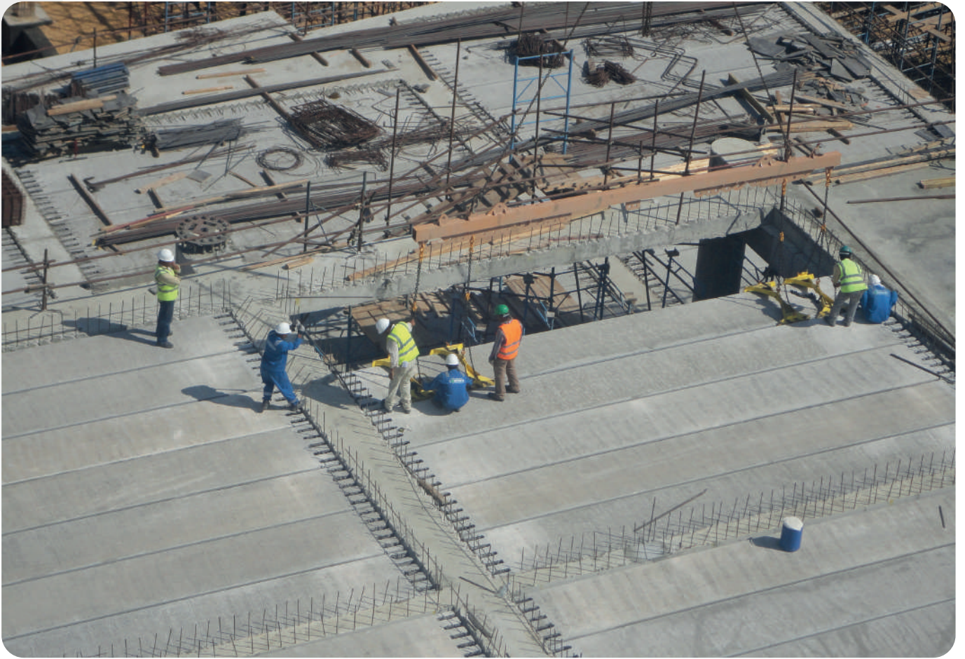
Hollow core slabs swift erection Cairo Airport - Cairo
