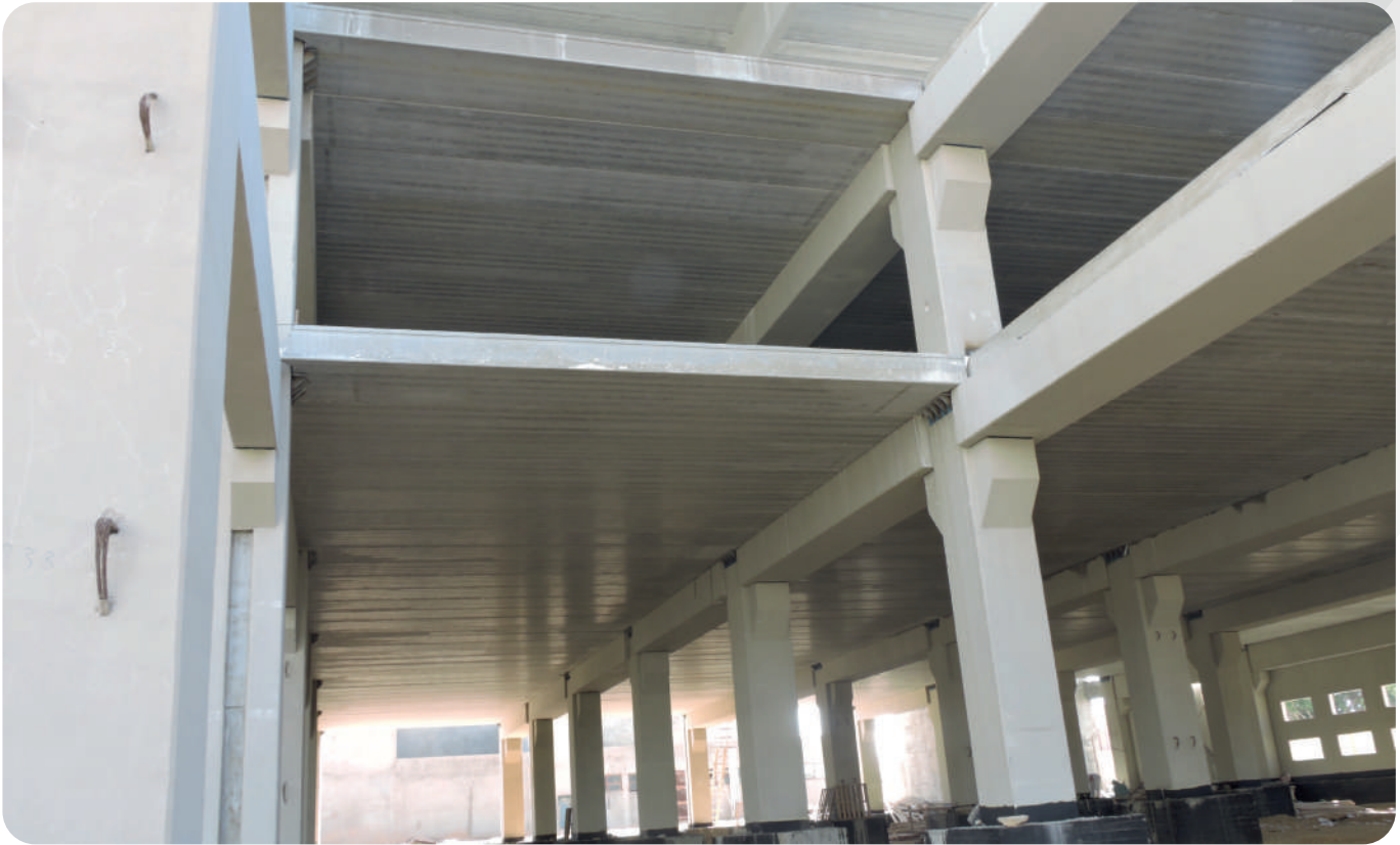
Hollow core slabs finish surface as per mold casting Fourtex Textile factory - Sadat City
