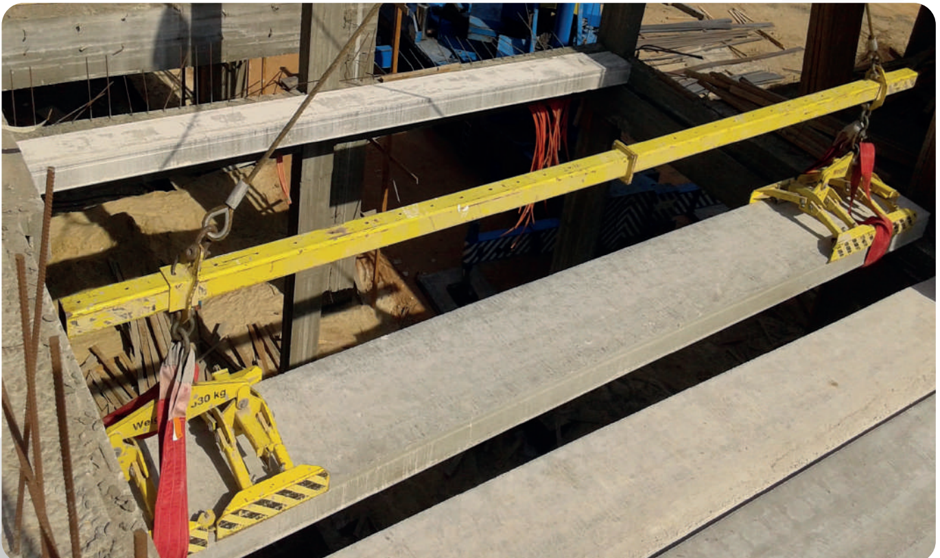
Immediate deck just after erection Noor EL-ELM international school - Sadat City
