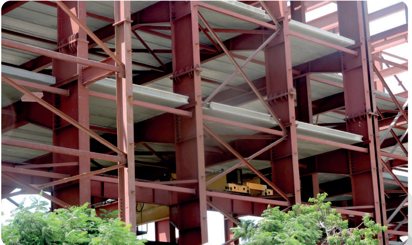
Covering Multiple stories without any formwork TOSHIBA ALARABY factory - Quesna city
