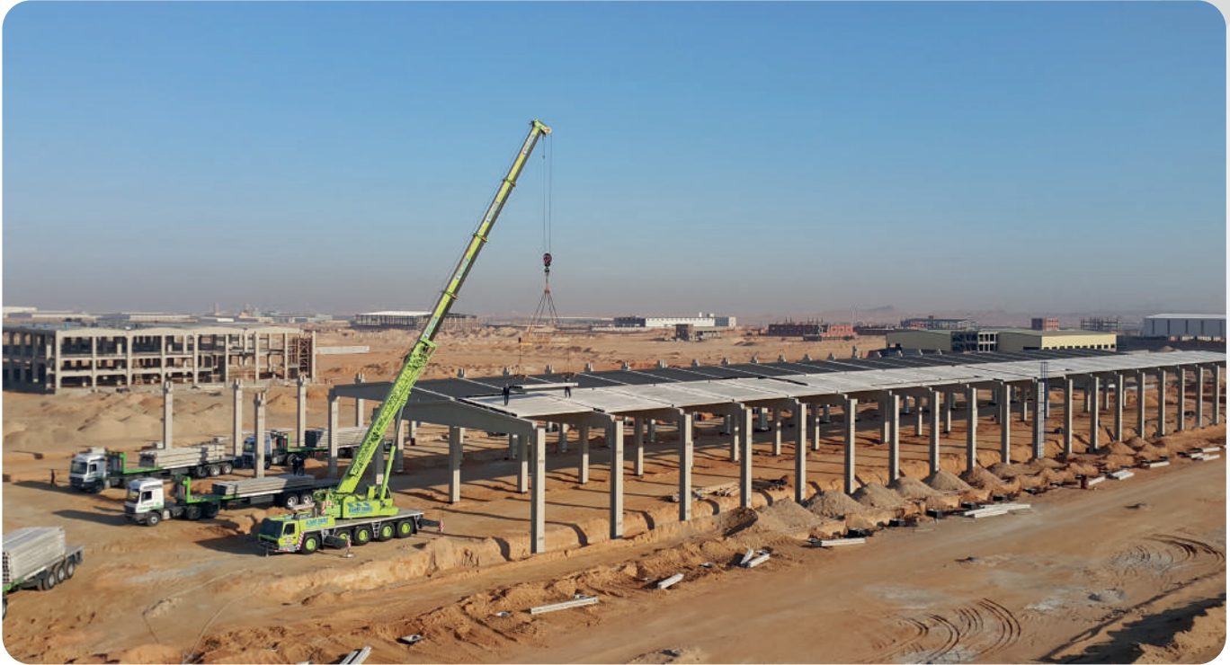
Hollow core slabs full package by Modern concrete Farag Textile factory - 10th of ramadan
