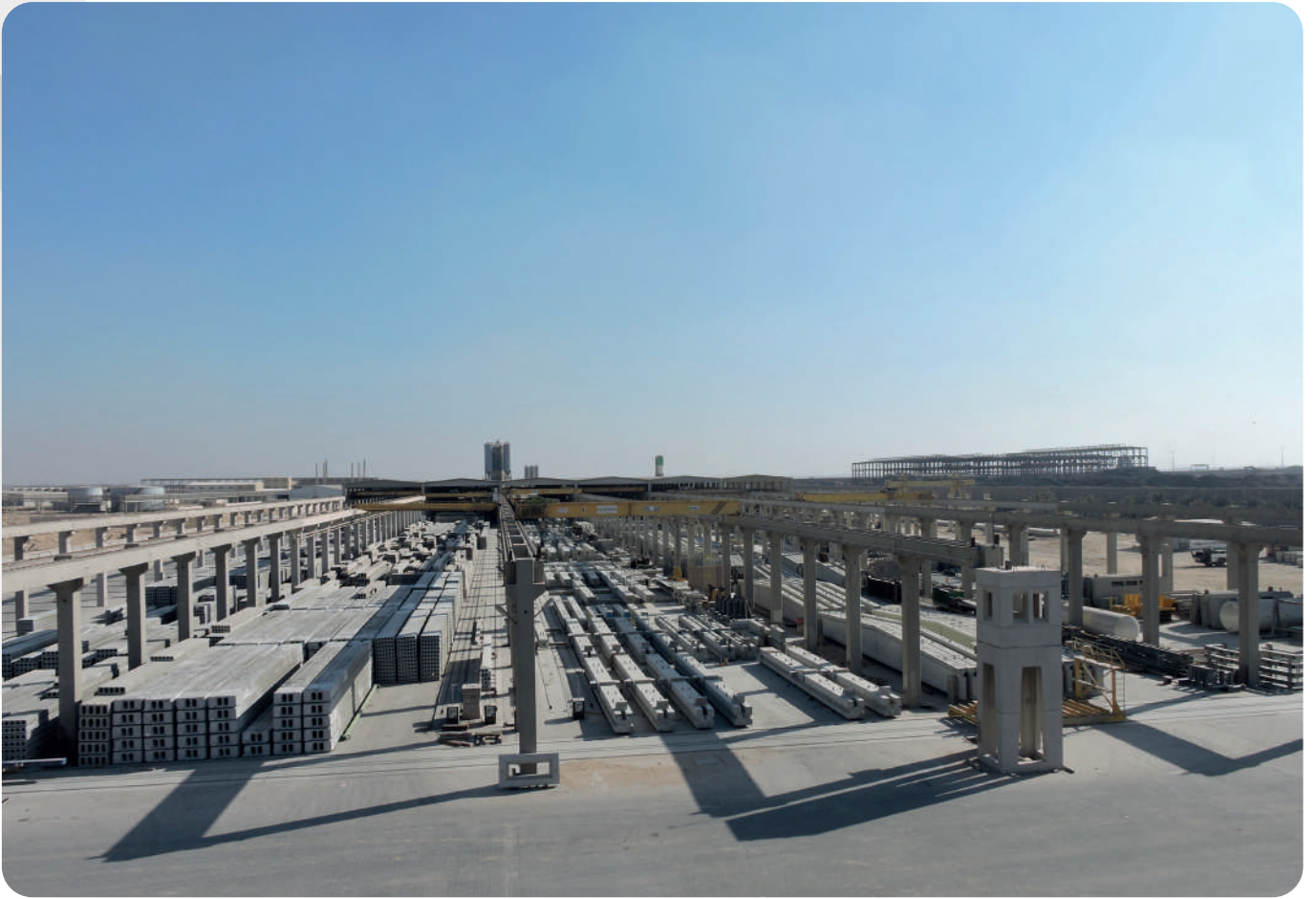
Stock Yard for Precast Concrete factory
