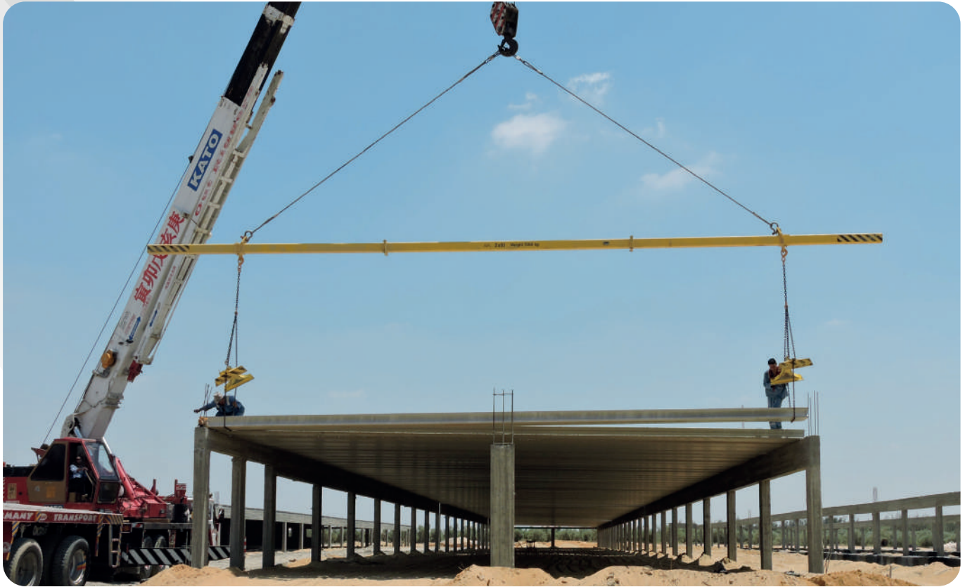
Covering long spans without any formwork ALWADI Poultry ward - AIWADI ALGADED
