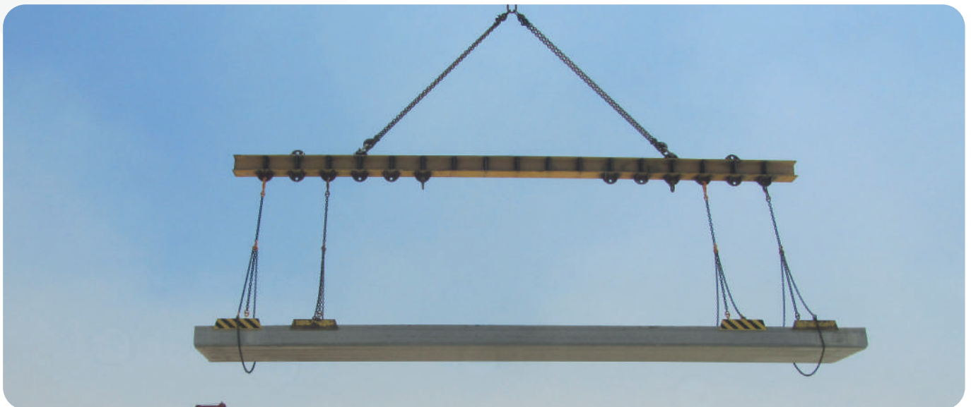
Hollow core slabs lifting using special spreader beam and clamps
