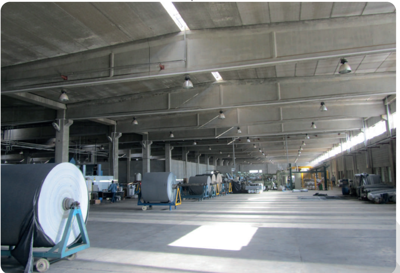
Hollow core slab gives wide spans Fourtex textile factory - Sadat City
