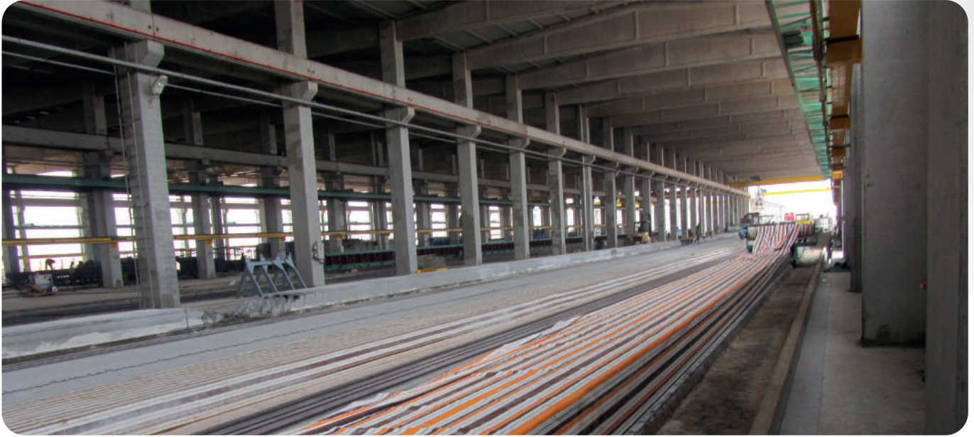
Covered bed for curing
