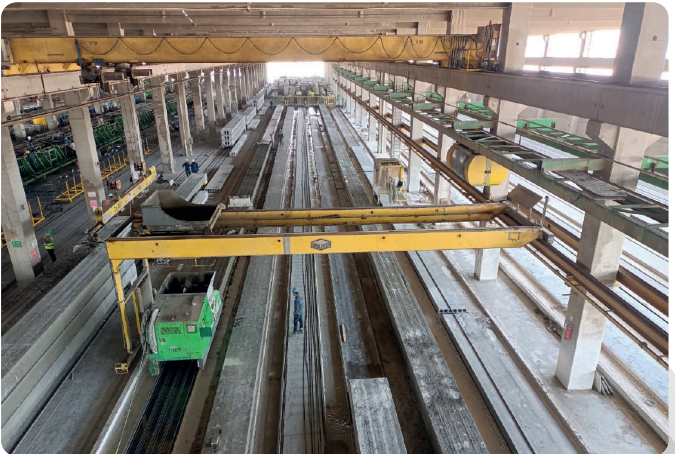
Hollow Core slabs factory
