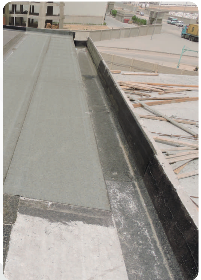
Applying the insulation sheets Baskolita factory - 6 October City
