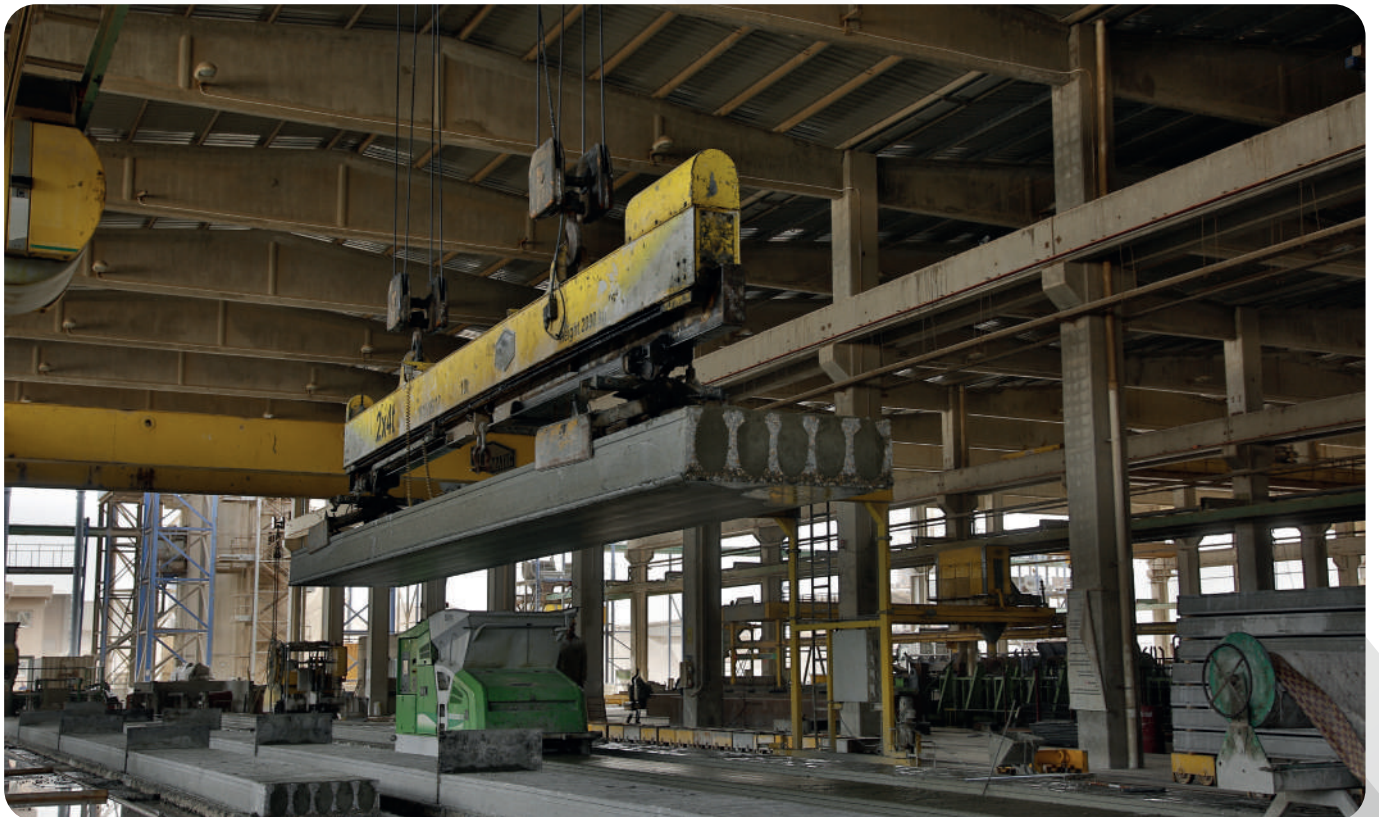
lifting Hollow core piece after cutting process
