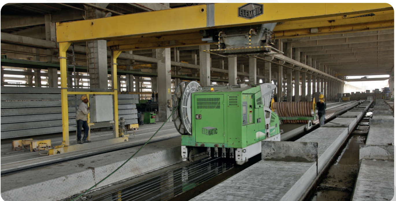
Strands cable lay-down
